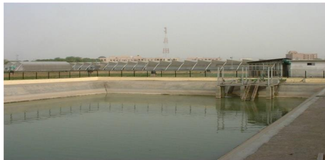
Fig 1: RCC Farm Pond/Reservoir Capacity 40,000 cubic meter
