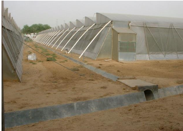
Fig 3: Greenhouse Roof Top rain Water Harvesting System with Drains
