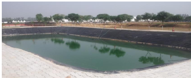
Fig 2: Geomembrane Lined Pond/Reservoir Capacity 40,000 Cubic Meter
