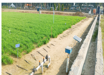
Automated sub-surface drip irrigation system
