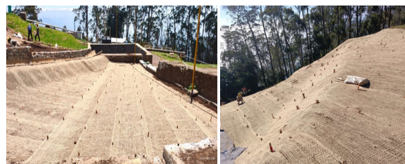
JGT is being laid out after backfilling the remediated soil
